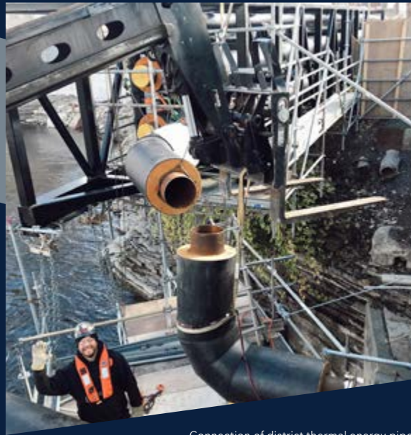
Connection of district thermal energy pipes
